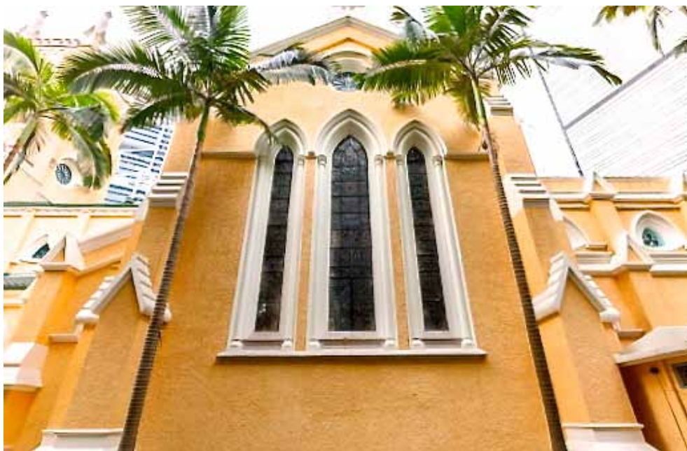
The South Transept looking 'cool' in its new colour scheme
